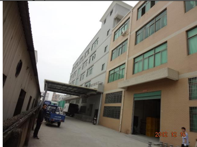
1. Factory out side view
