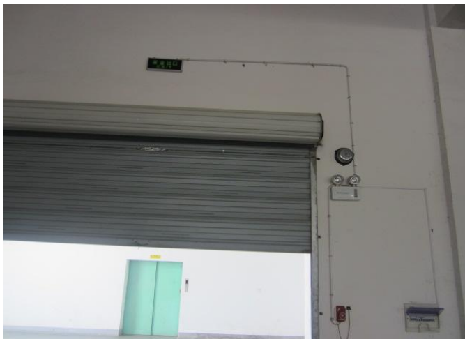
Exit and fire alarm
